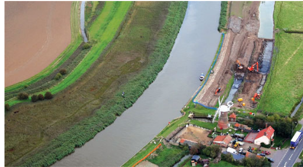
Working on flood banks, Broadlands, England
