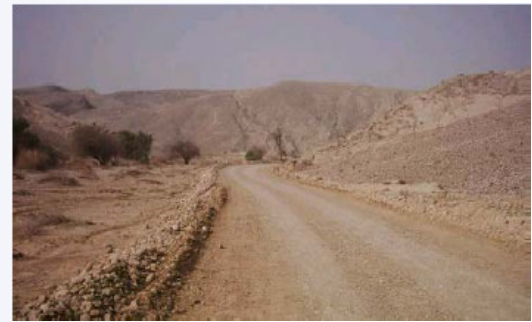
Gravel Access Road track-Mehar 2 Well, Sindh, Pakistan
